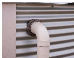
100mm Overflow for Steel Liner Tank
