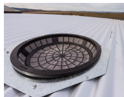
500mm Leaf Sieve for Steel Liner Tank
