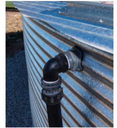
50mm Inlet for Steel Liner Tank
