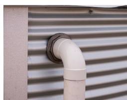
100mm Overflow for Steel Liner Tank
