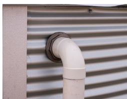
100mm Overflow for Steel Liner Tank
