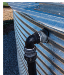
50mm Inlet for Steel Liner Tank
